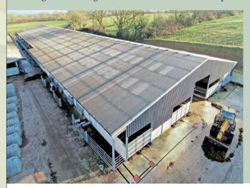
six-inch corrugated profile, which is the perfect match for traditional asbestos. "This is not only important from an aesthetic point of view, but also simplifies the fixing process," says the company's Ged Ferris.
