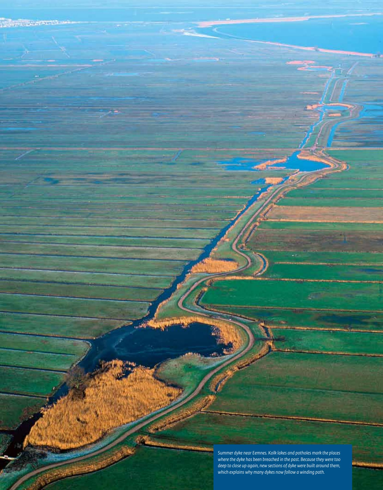
Summer dyke near Eemnes. Kolk lakes and potholes mark the places where the dyke has been breached in the past. Because they were too deep to close up again, new sections of dyke were built around them, which explains why many dykes now follow a winding path.
