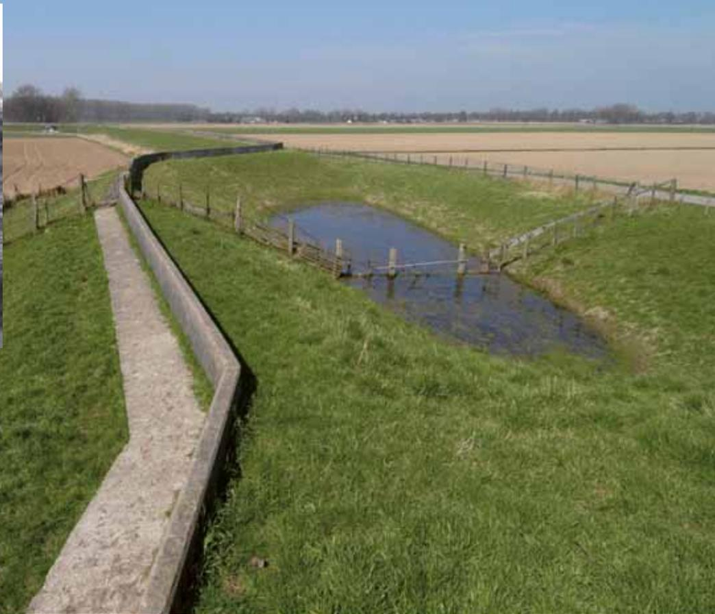
*Muralt wall on the Schenkeldijk at Werkendam. Countless dykes in Zeeland were reinforced with these walls between 1906 and 1939. Most have since been removed.*
