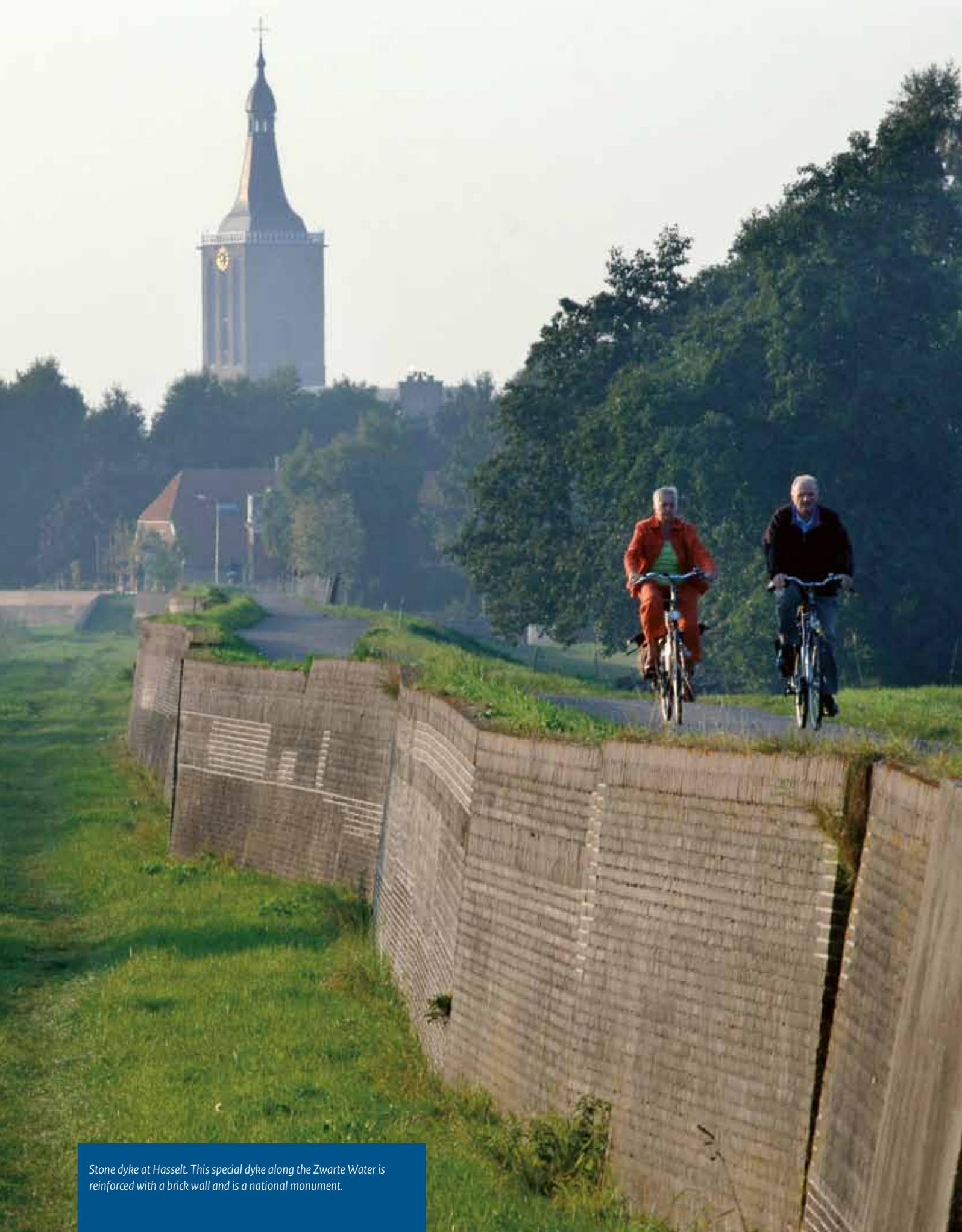
Stone dyke at Hasselt. This special dyke along the Zwarte Water is reinforced with a brick wall and is a national monument.
