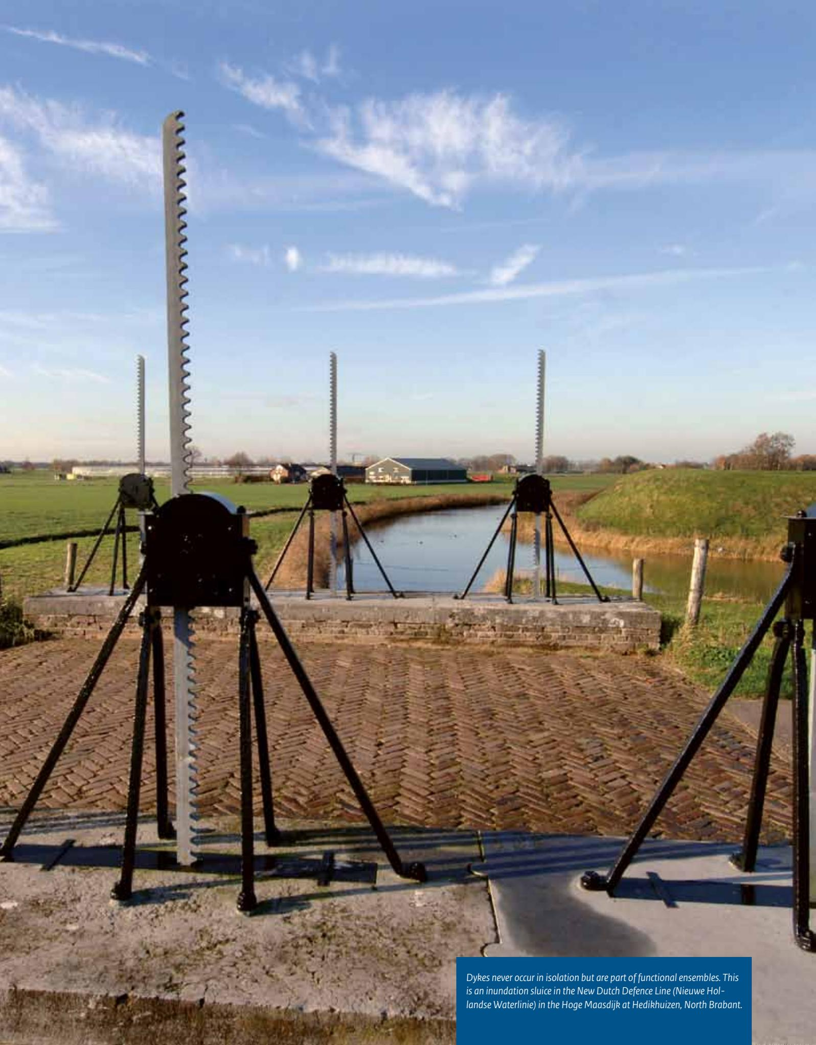
*Dykes never occur in isolation but are part of functional ensembles. This is an inundation sluice in the New Dutch Defence Line (Nieuwe Hollandse Waterlinie) in the Hoge Maasdijk at Hedikhuizen, North Brabant.*
