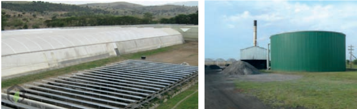
Figure 32. Solar collector for greenhouse heating (left; www.certhon.com ) and a heat storage tank (right).
