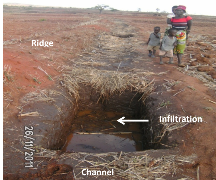
Figure 2.3: A contour ridge with infiltration pits Rushinga district Zimbabwe
