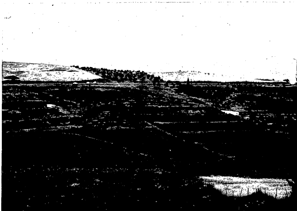
Figure 18.2 Panorama of a bench terraced valley slope under gravity irrigation. Note that every individual landowner used different methods and specifications for the construction of the terraces. Step heights vary from 1 to several meters. Some terraces were made by mule drawn ploughs. The main tendency is for large step heights which require heavy machinery.
