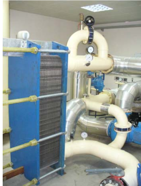
Figure 1.2. A plate heat exchanger that separates the geothermal water from heating system water that circulates in the heating system of a greenhouse (photo taken near Dikili).
