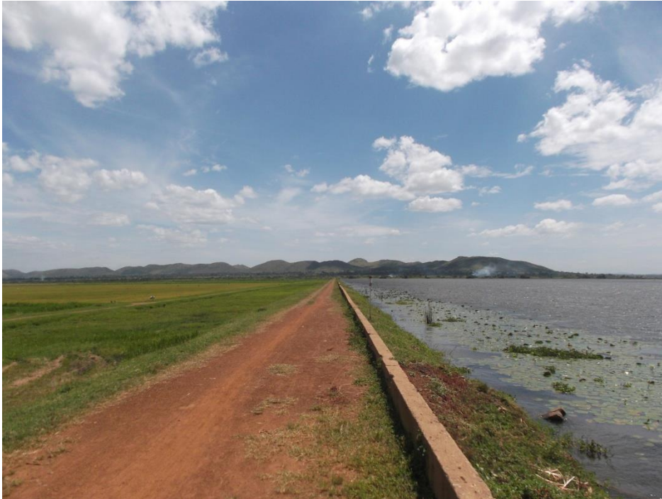
FIGURE 3, THE DAM OF THE KIBIMBA RICE IRRIGATION SCHEME
