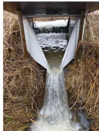
Figure 4.4: The weir installed at the Gryteland catchment. Picture taken during fieldwork spring 2013. Photo by: Torsten Starkloff.
