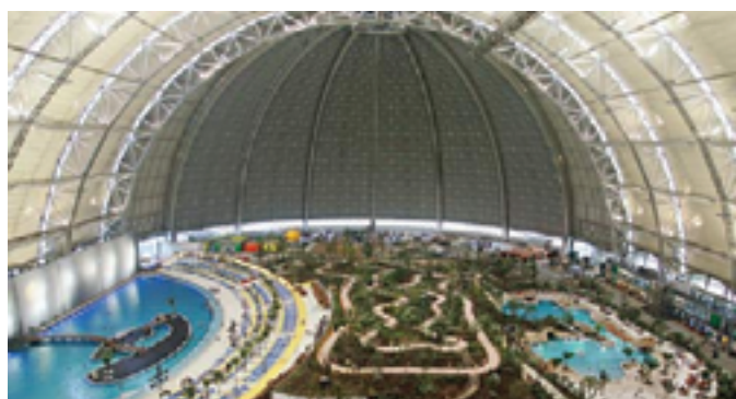
6.36 Several swimming pools can be found in the hangar (Lowara)
