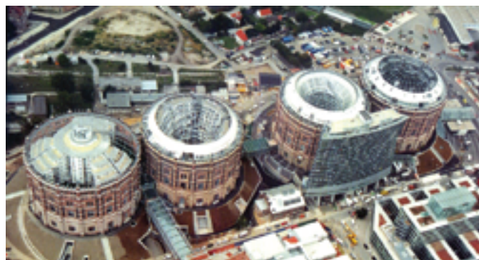
6.26 Gasometer City (adaptivereuse.info)
