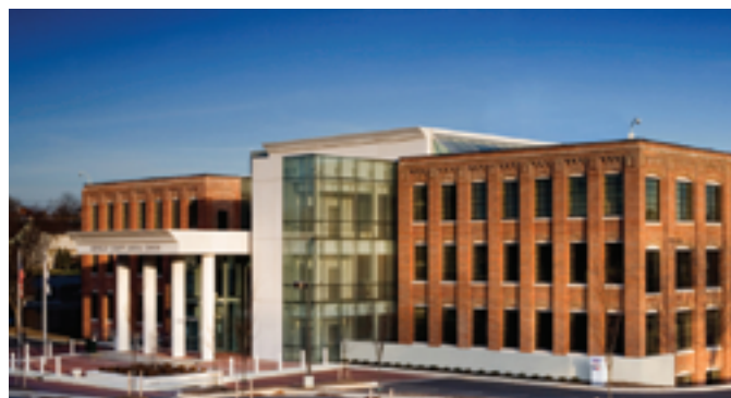
6.22 Berkeley County Judicial Centre (adaptiveuse.info)
