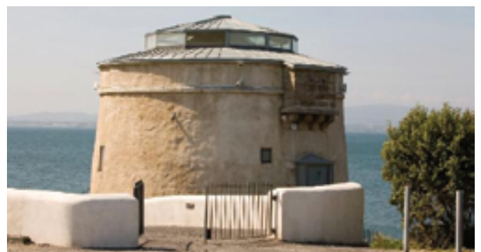
6.44 The Martello Tower at Sutton (Martello Tower Sutton)
