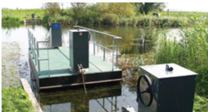
7.13 A pull ferry as a way to enter the fortress as a pedestrian (Henk v.d. A)
