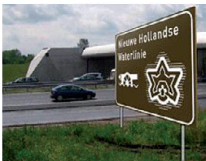
1.1 Signs have been placed along the highway to make people more aware of the location of the New Dutch Waterline in the landscape
