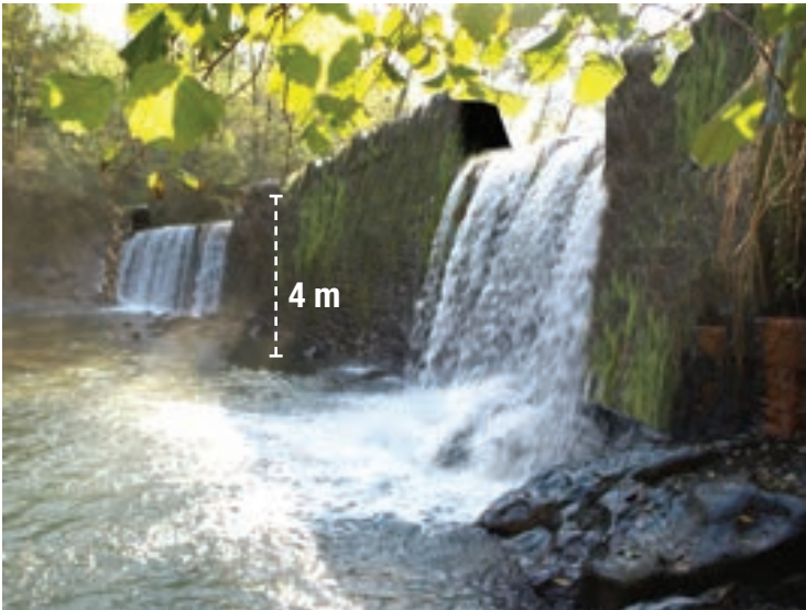
[15.5] By heightening them in the form of orifice dams up to 4 meters retention capacity is created
