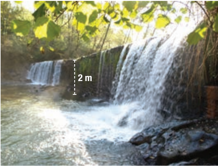
[15.4] The ferreria dams have a height of between 2 and 3 meters in the current situation
