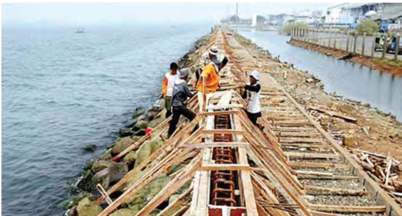
Figure 3. 8 Construction of a dike to reduce fl ooding from high tides and extreme waves in East Harbour of Muara Bary, Jakarta. (Source: Media Indonesia, 2007 in ISNC)
