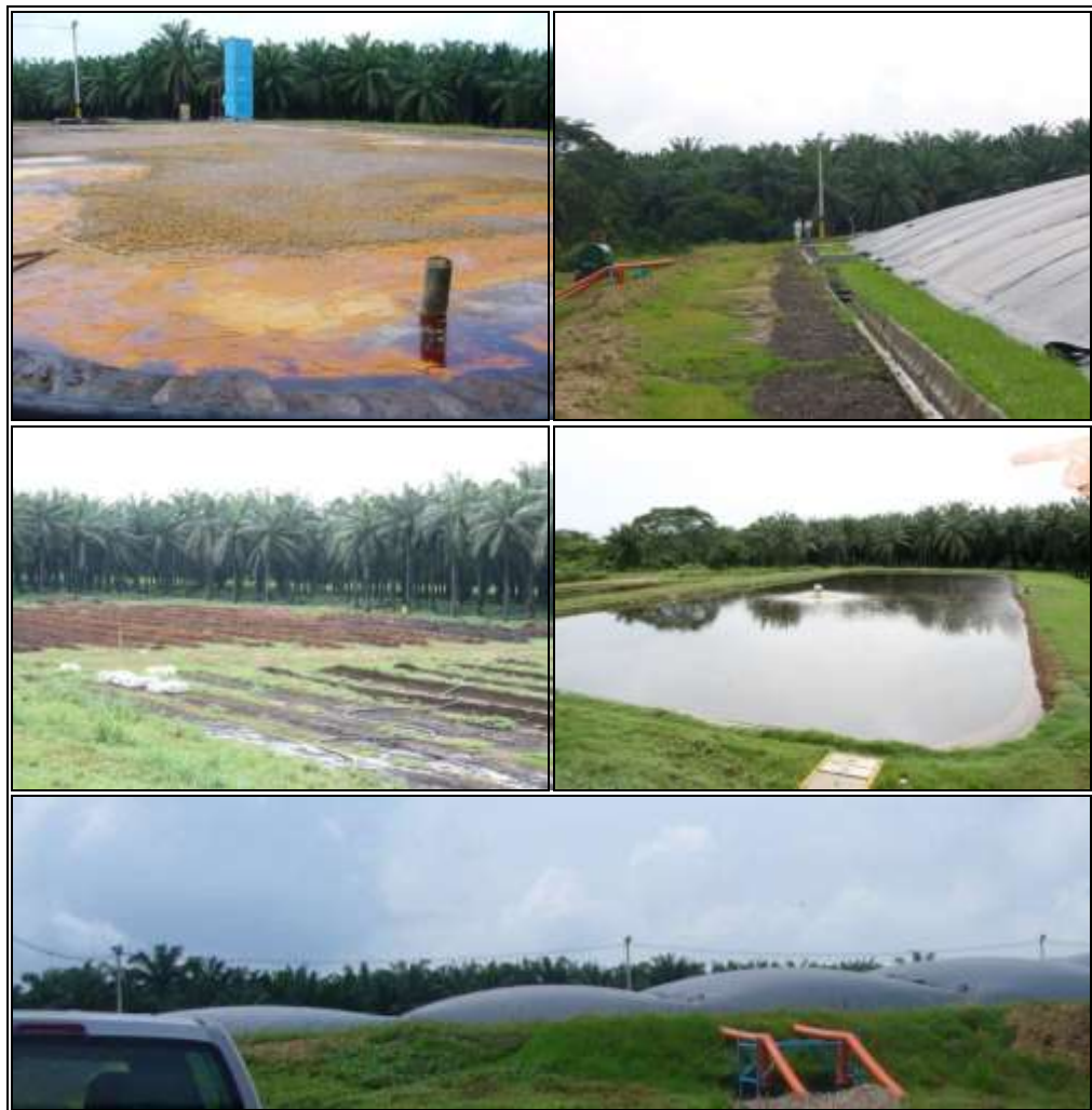
Figure 8. Palm oil mill effluent is cooled down before being transferred into the tarp covered biogas reactor. The sludge is used to make compost and the effluent is also returned to the plantation after aerobic treatment. (Pictures taken at Tequendama plantation in Colombia).
