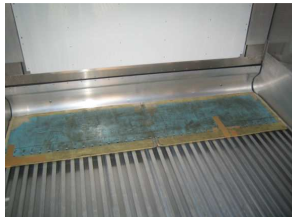
Fig. 13, plating covering first 50 cm of T-bar for air circulation measurement (step 7 above).
