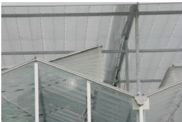
Figure 6.3. Insect nets in the window opening of a Venlo-type greenhouse, combined with an external shading screen
