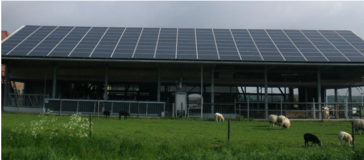
Figure 6.4. A dairy farm in The Netherlands using a Grid -Tie system with solar panels on the roof. Source: (Author, 2013)
