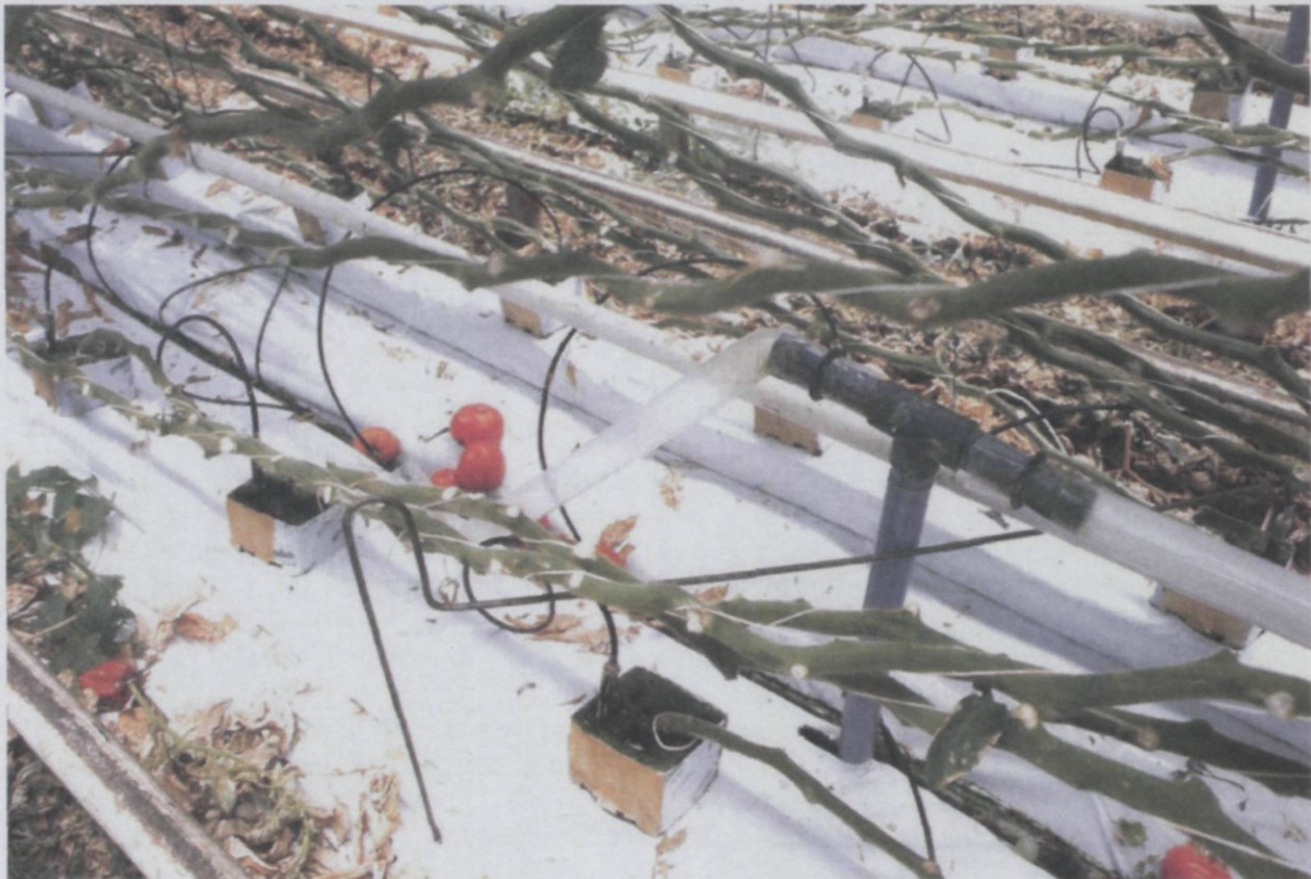
Distribution system for CO 2 with hoses pinched by stems or fruits because the pressure in the hoses is too low
