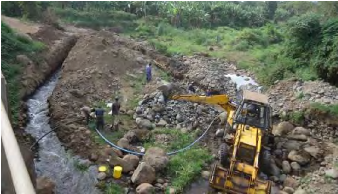
Figure 3 - groundwater pipe construction (source: field observation 1-12-2012)
