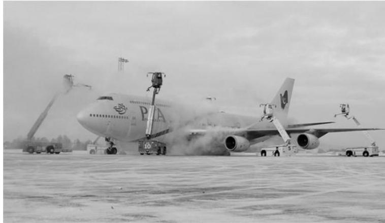
Figure 1.1: Spraying of de-icing chemical (picture: OSL).
