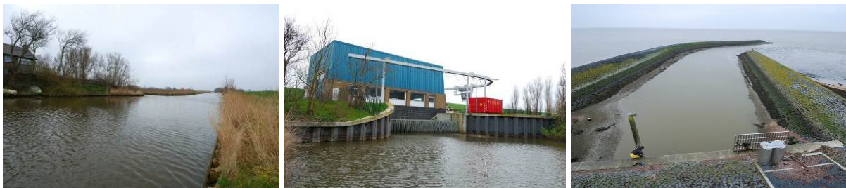
Figure 3.1.3. Ropta; the canal leading to pumping station Ropta (left), pumping station (middle) and the canal behind the pumping station leading to the Wadden Sea (right).
