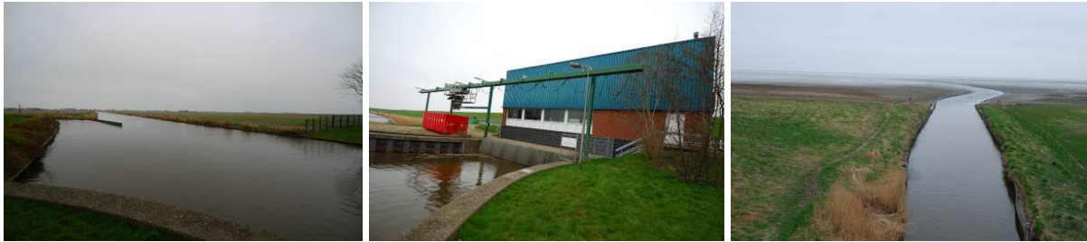
Figure 3.1.2. H.G. Miedema; the canal in front of the pumping station (left), pumping station (middle) and the canal behind the pumping station leading to the Wadden Sea (right).
