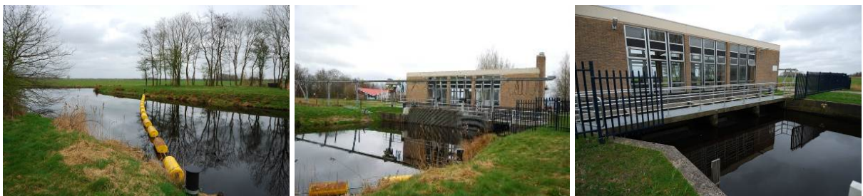
Figure 3.1.5. Offerhaus; the canal adjacent to the pumping station (left), pumping station (middle) and the rear of the pumping station (right).
