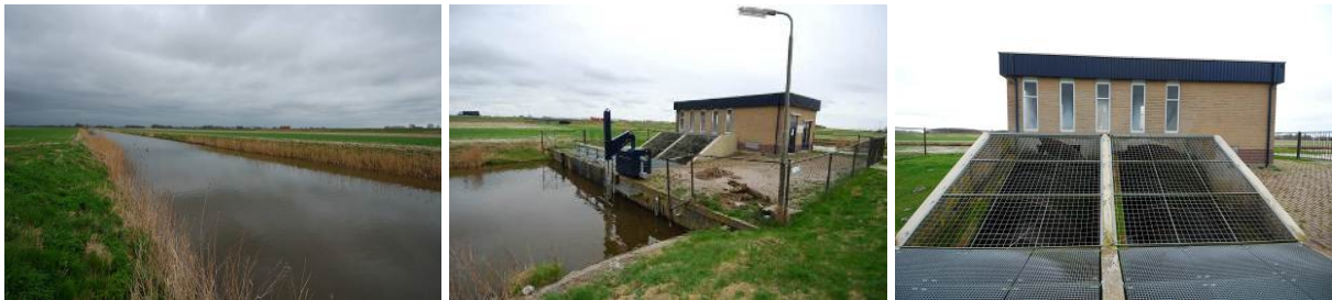
Figure 3.1.4. Schalsum; the canal in front of the pumping station (left), pumping station (middle) and the pump blades (right).
