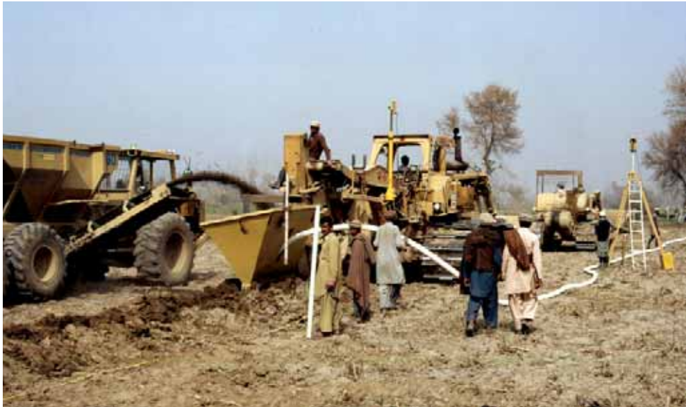
Figure 7 Trenchless drain installation in the Mardan SCARP project area
