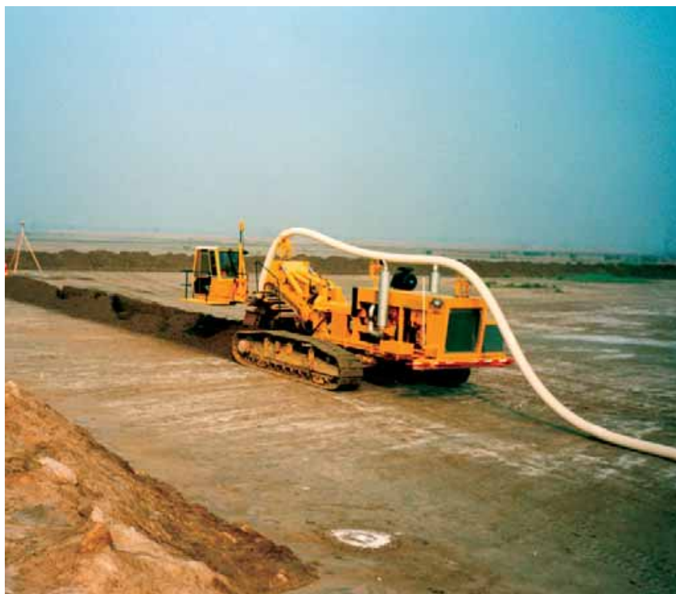
Figure 4 Trencher machine installing a plastic collector drain in North-West China
