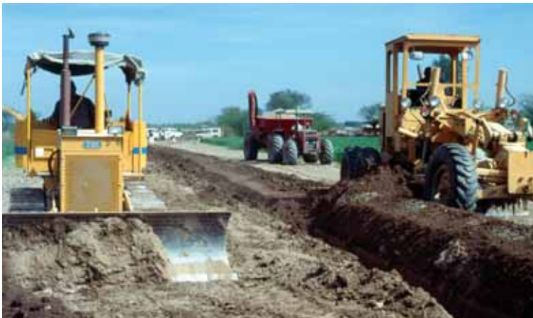
Figure 59 Backfilling of the drain trench: using a dozer and grader
