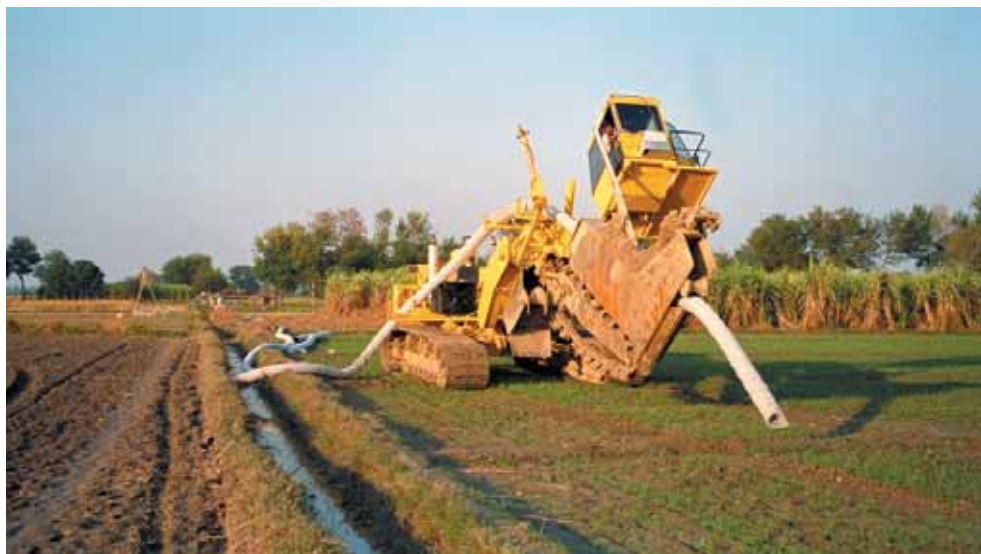
Figure 7 Trencher installing pre-wrapped corrugated drain pipe in Gohana area
