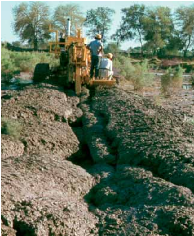
Figure C24.2 Trencher operating in unstable soil
