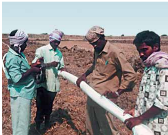
Figure 8 Wrapping of envelope material (nylon mesh) around the pipe in Uppugunduru Pilot Area, Andhra Pradesh
