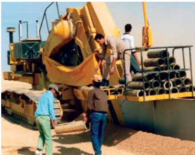
Figure 14 A rock trencher installing a concrete collector drain operating in the Nubaria area
