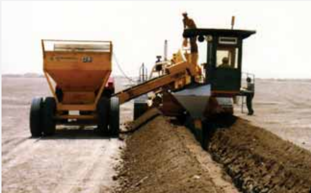
Figure 57 When the gravel is placed manually, the drain pipe easily gets dislocated (a), when gravel is applied through a gravel box mounted on the trench box of the trencher the drain is not dislocated (b)
