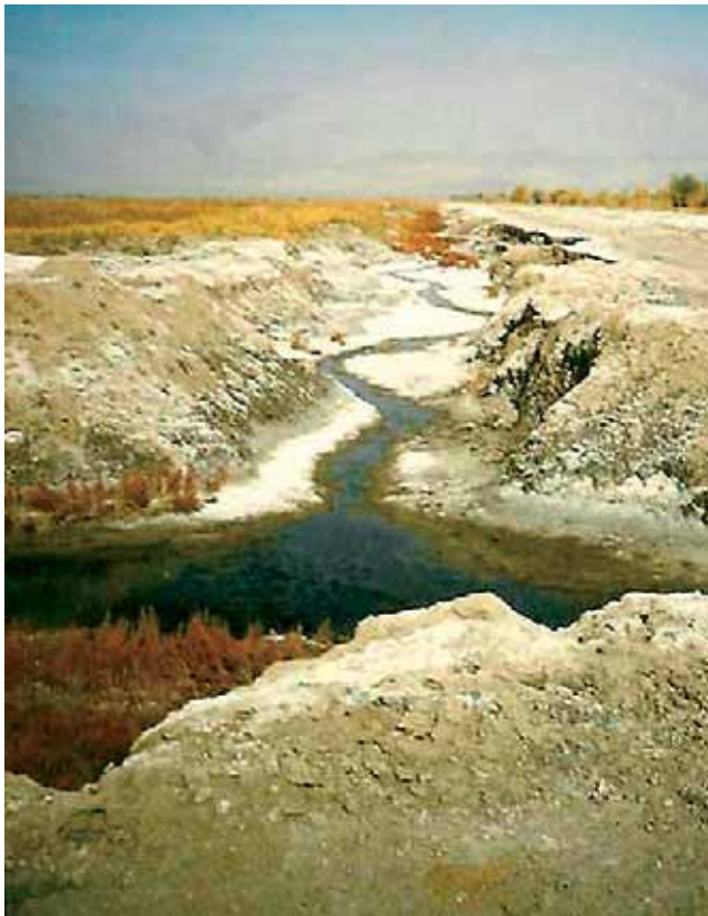
Figure 3 In the unstable soils of North and North-West China open drains are not very sustainable
