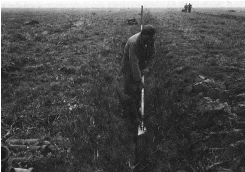
Figure C36.3 Digging a drain trench by hand
