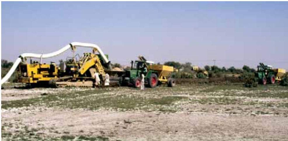
Figure 6 Installation of large diameter perforated corrugated PE collector drain pipe with gravel envelope
