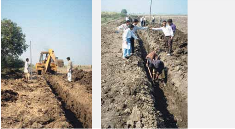
Figure 50 The combination of mechanical and manual installation consists of digging the drain trench with a hydraulic excavator and placing the drain pipes into the trench by hand (Example Segwa Drainage Pilot Area, Navsari, Gujarat, India, for more details see Part III)
