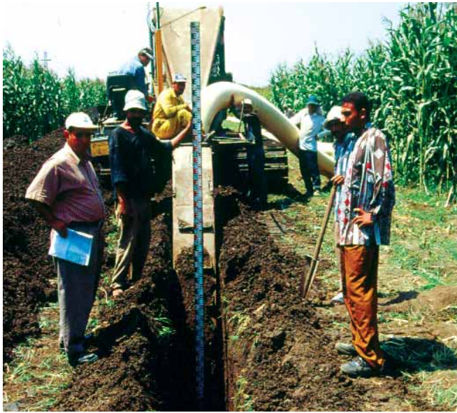
Figure 15 Installation of large size corrugated PVC pipe
