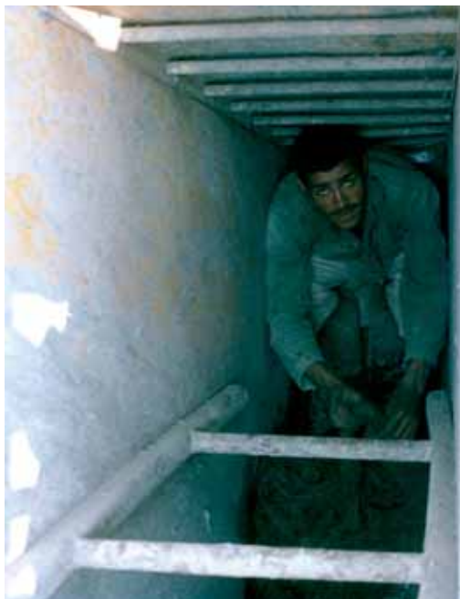
Figure C23.5 A labourer in the trench box to put cloth around the joints
