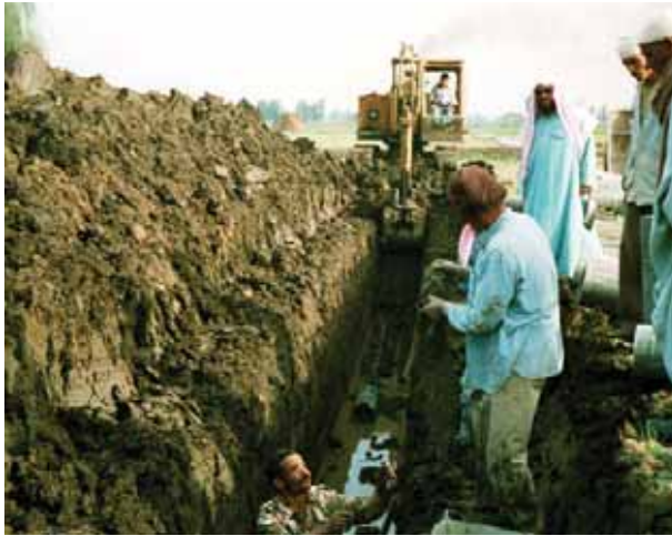
Figure 32 Hydraulic excavator digging a drain trench
