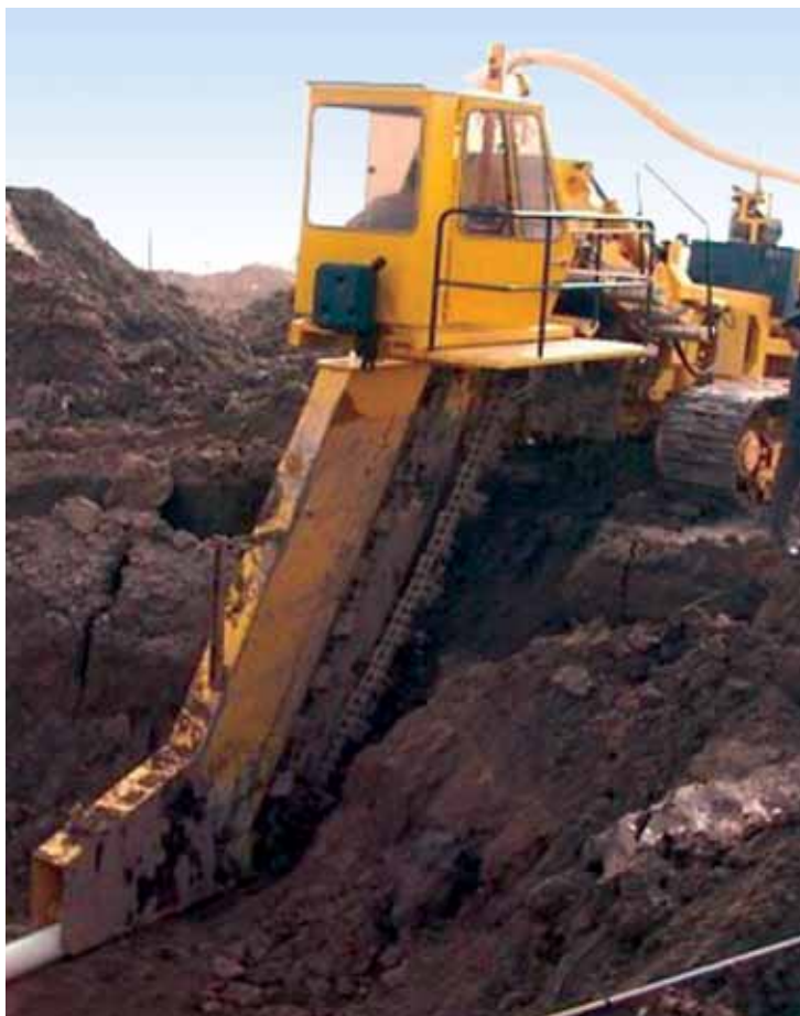
Figure 6 Installation of a collector pipe in North-West China
