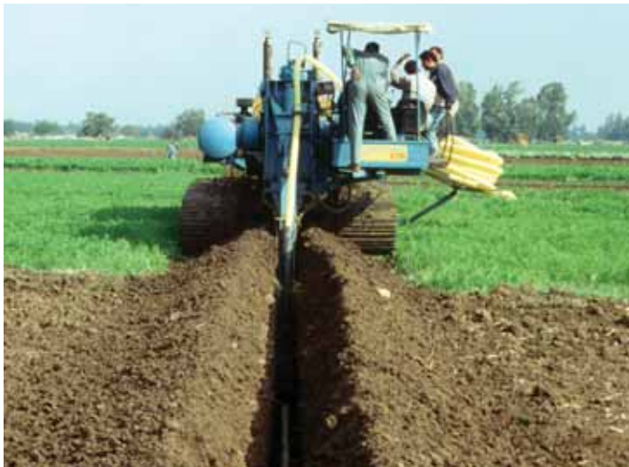
Figure 55 Excavating the trench
