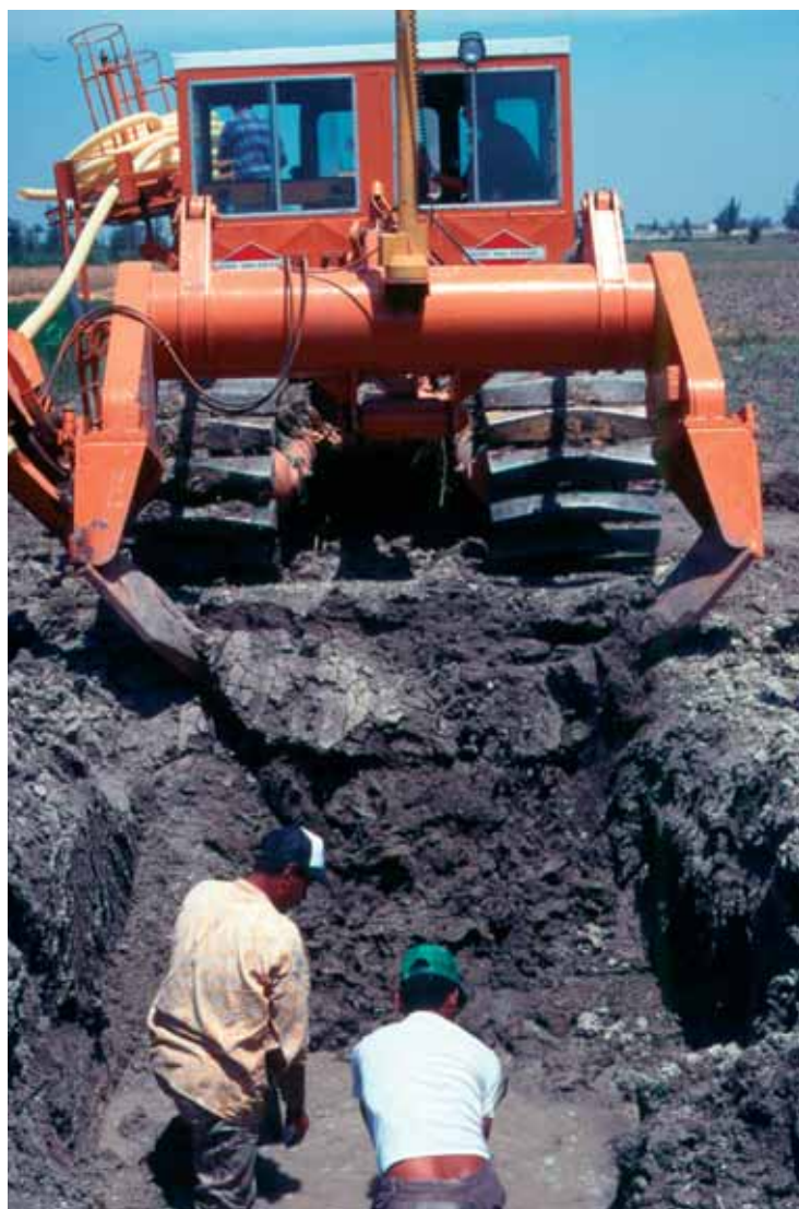
Figure C12.3 V-plough starting the installation of a field drain at the collector drain (composite drainage system)
