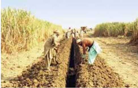
Figure C33.3 Blinding/backfilling the trench by hand
