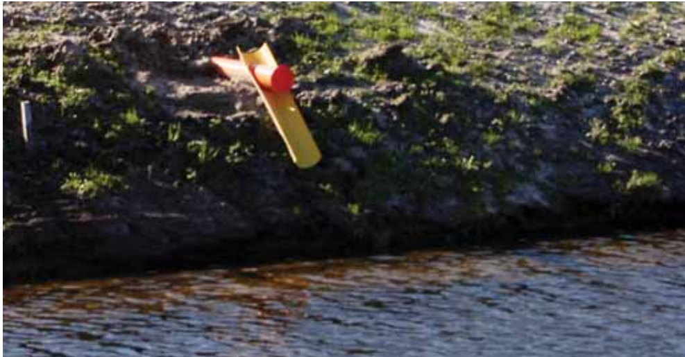
Figure 8 End chute to protect the side slope of the open collector drain against erosion
