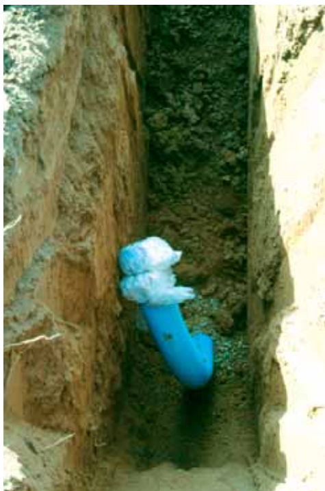
Figure C23.2 Plugged end of field drain
