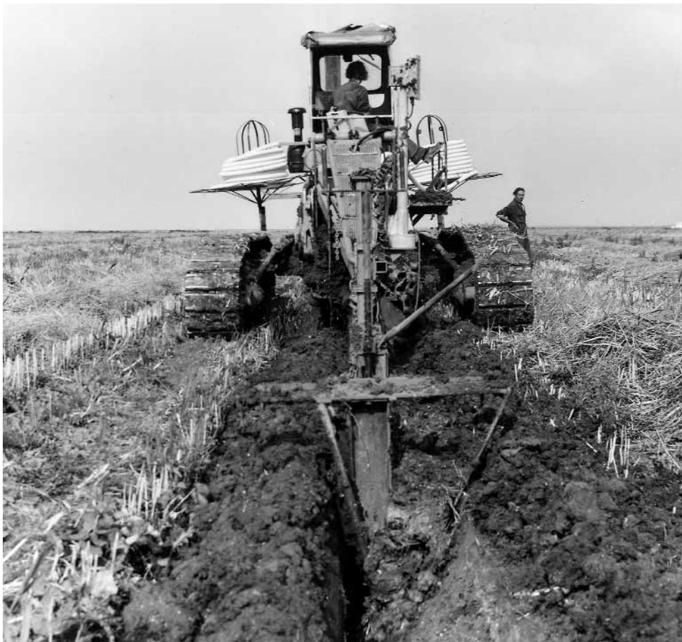
Figure 10 Trencher operation in reclamation area with blinding knife at the trench box
