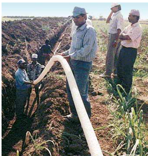
Figure 9 In Segwa, the drain trench was excavated mechanically and all other activities were done manually: a) excavating the trench; b) checking the level; c) preparing the bed; d) checking the final level; e) checking the level at the outlet and f) laying the pipe
