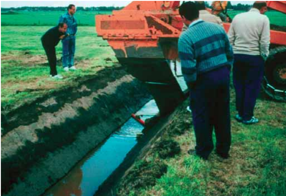
Figure C12.1 V-plough starting installation of a field drain from an open drain
