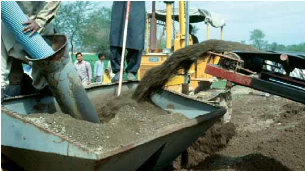
Figure C35.2 Unloading of gravel trailer into the hoppers of the trencher
