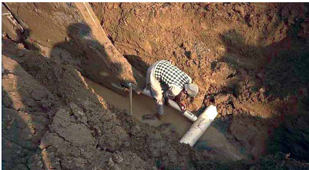
Figure 2 Before the field drains are installed, the field drain is connected to the collector drain using a plastic T-joint
