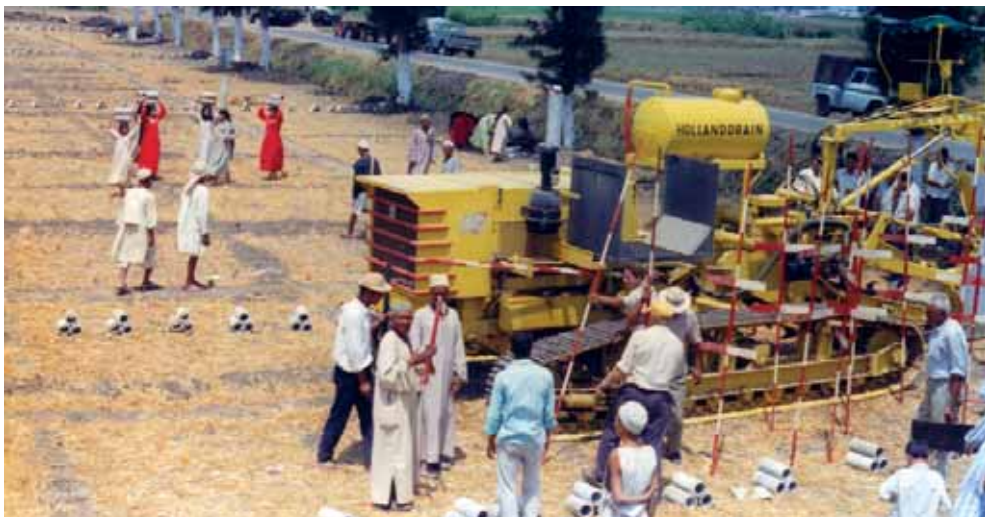
Figure 3 Mechanical installation of subsurface drainage was introduced in Egypt in the 1960's
