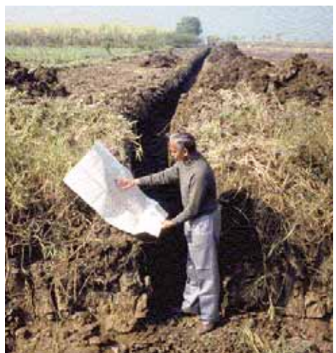
Figure 9 In Segwa, the drain trench was excavated mechanically and all other activities were done manually: a) excavating the trench; b) checking the level; c) preparing the bed; d) checking the final level; e) checking the level at the outlet and f) laying the pipe
