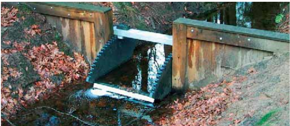
Figure 3 Fixed (a), adjustable (b) and movable (c) weirs are used to maintain the water level in the open drainage system at the desired level
