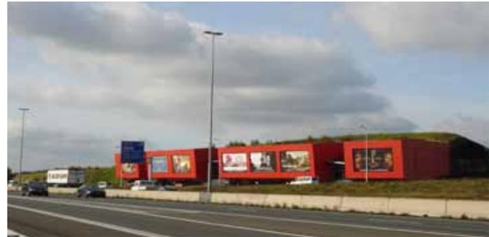
Architecture integrated into highway noise barrier
