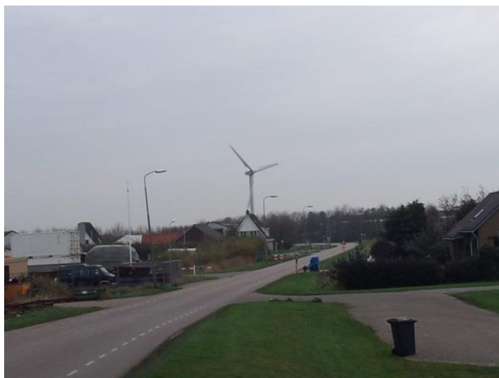
Fig. 16 The only (large) wind turbine of Texel
