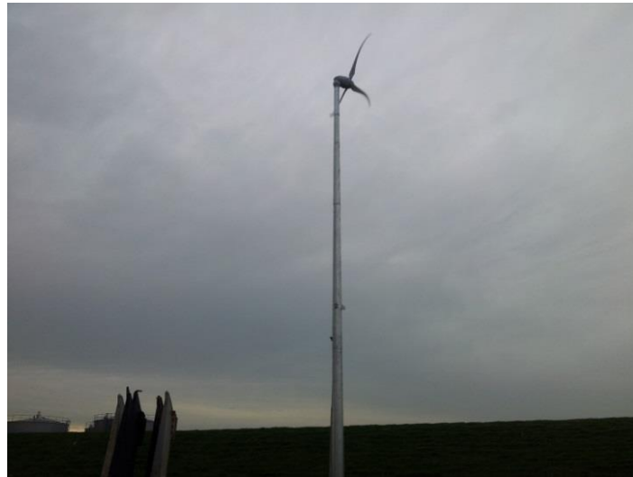
Fig. 13 Small wind turbine at 't Horntje
