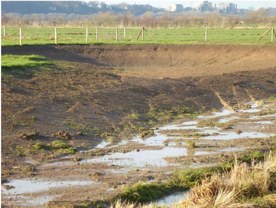
Figure 15: Construction of a pool and swamp banks on the northern border of the farm.
