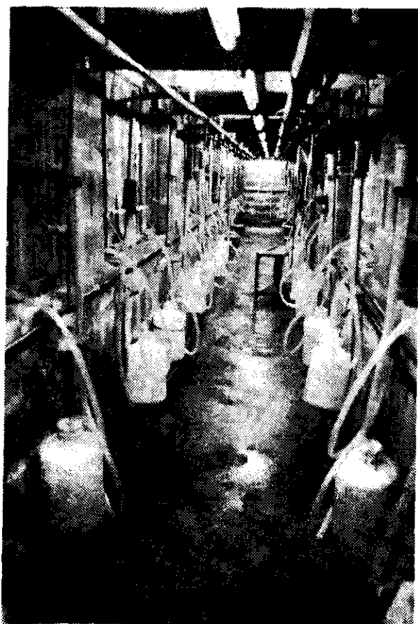
Fig. 9. Detail of the tunnel for regulation of water tables, collection of drainage water, sampling the soil and monitoring soil temperature
