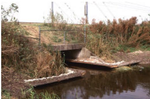
Figure 10. Walking strips in a culvert provide connectivity for migrating small mammals between habitat patches bisected by infrastructure (Photograph: Edgar van der Grift)
