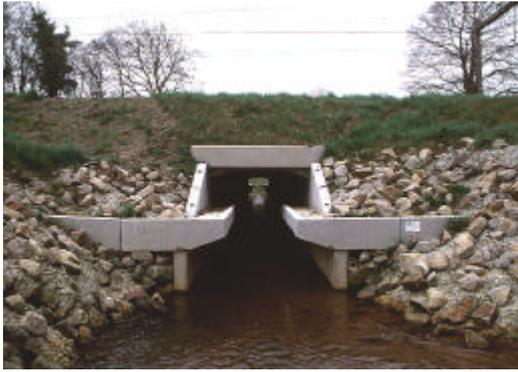
Figure 8. Ledges on both walls of a culvert enables newts to pass infrastructure (Photograph: Edgar van der Grift)
