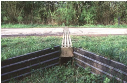
Figure 7. Small fauna underpasses proved to be effective means to help amphibians cross roads safely (Photograph: Edgar van der Grift)
