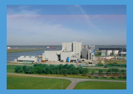
Poultry manure incineration 400.000 t/year, 36 MWe 25 % phosphate in ash Nitrogen & organic matter lost Subsidized...
