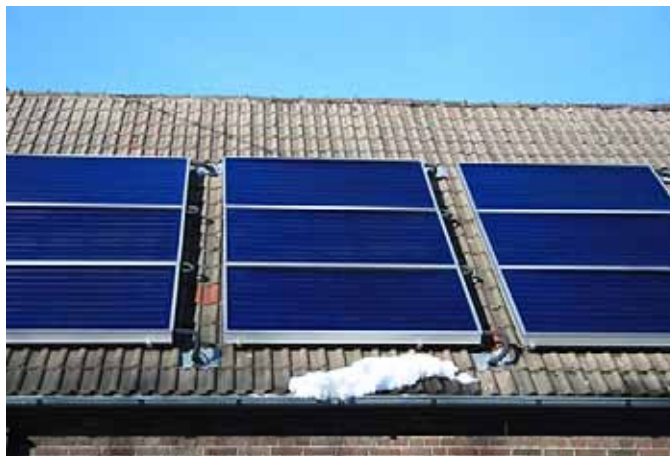
Solar water heater (left)
