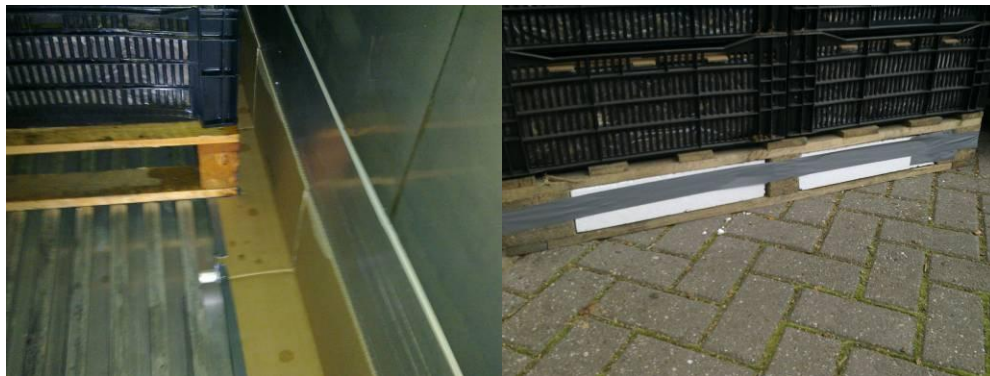
Figure 6: cover at right side of first 6m of the container (left); filled up pallet opening (right).
