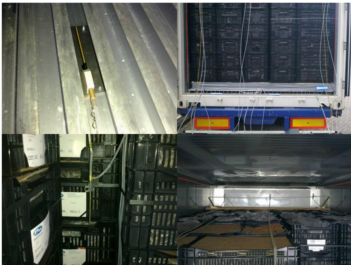
Figure 4: clockwise starting upper left: pitot tube in T-bar; pitot tubes in T-bar at 3 positions; 3 pitot tubes at sledge above the crates; pitot tube fixed in chimney.
