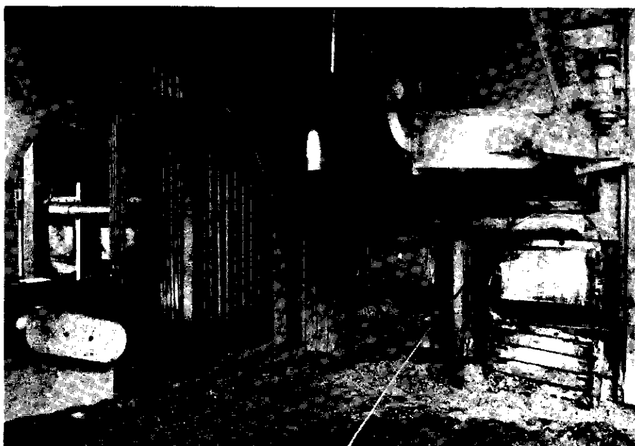
Plate 15. Steam boiler for fibre and nut shells.
