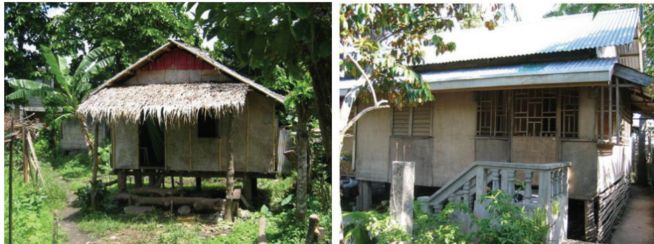
Figure 5.4 Elevated houses as a strategy to minimise exposure to flooding
