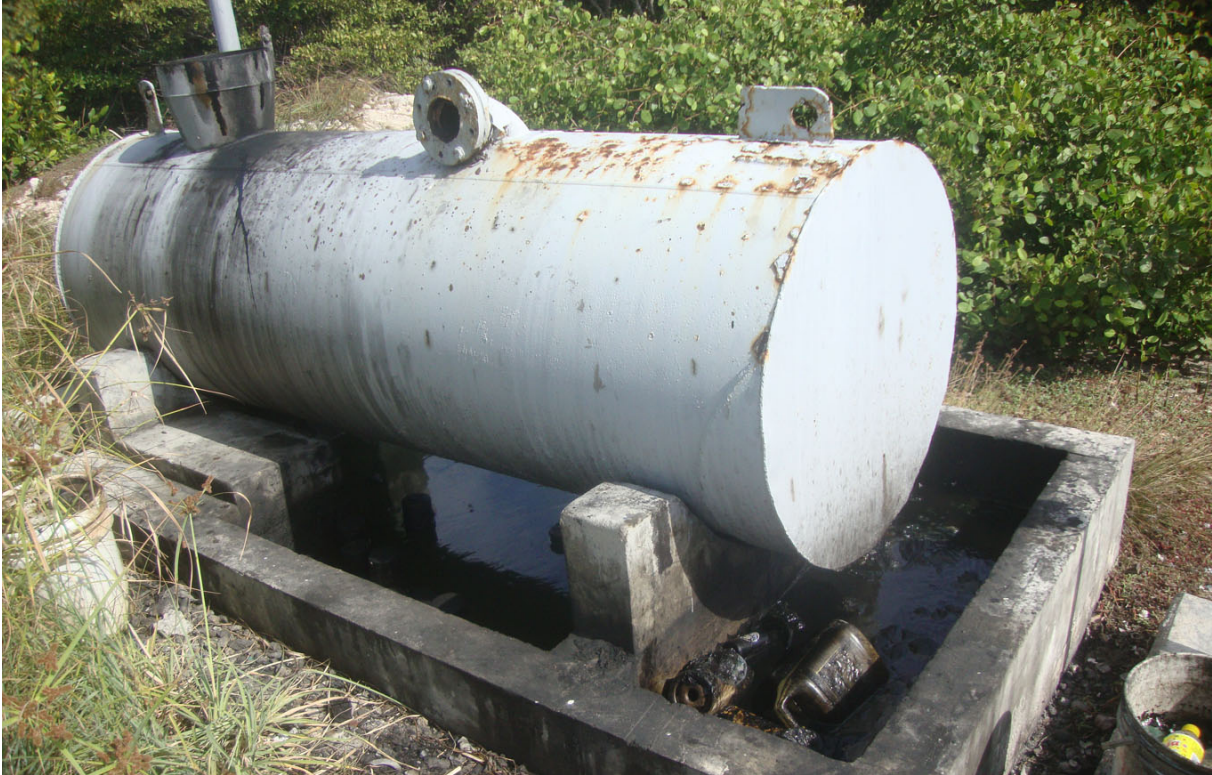
Fig. 9. Tank for collecting used oil from the fishing vessels docked at Sorobon, Lac.
