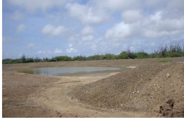
Fig. 6. Dam collecting rainwater.
