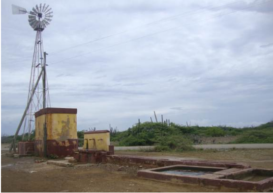
Fig. 5. Well driven by a windmill.
