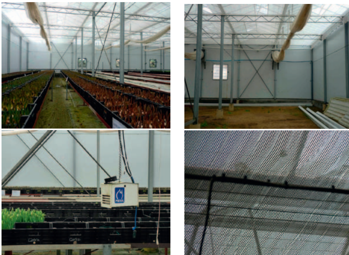
Figure 3.6. Construction elements in the high-tech greenhouse of Prominent Tulips at Rawsonville, in the Western Cape. Above left: tables with tulips and air outlet with fans; above right: air inlet and air hose; below left: measurement box of Priva; below right: light filtering screen.
