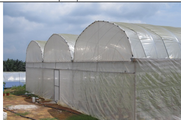
Figure 5.7: Fully closed greenhouse in Asia with no ventilation (very high temperatures inside)
