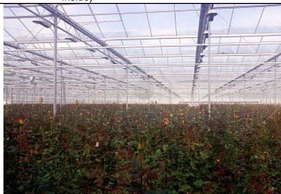
Figure 5.10: High-tech Netherlands greenhouse with assimilation lights
