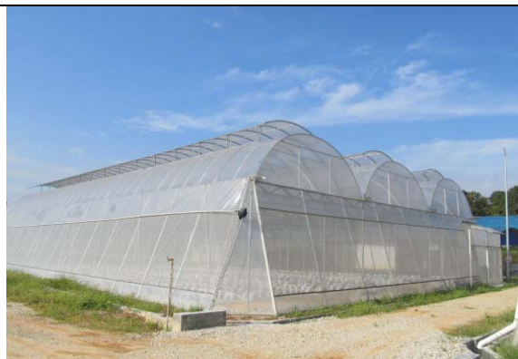
Figure 5.8: Greenhouse in Malaysia with side and chimney ventilation (good temperatures inside)
