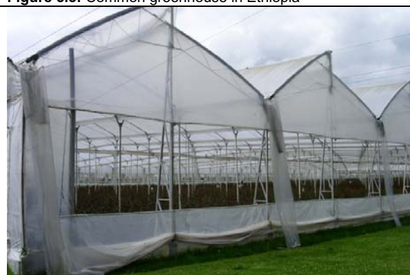
Figure 5.5: Greenhouse in Colombia with open sides and fixed open top covers
