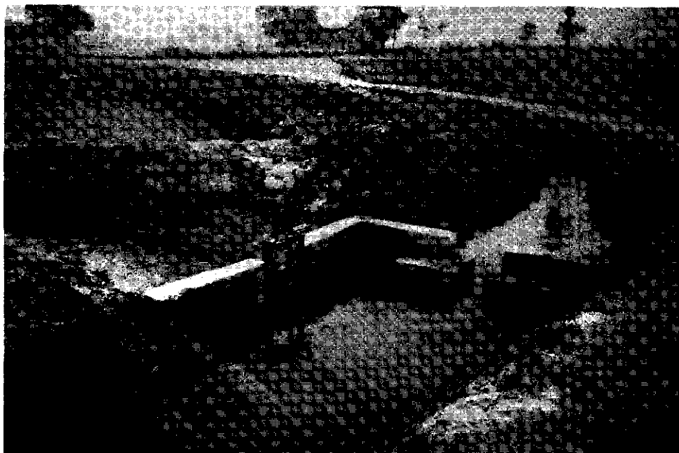
Photo 5.1 Concrete water division structure within a tertiary unit in Blocks 1 and 2 of MIP-I (1993)
