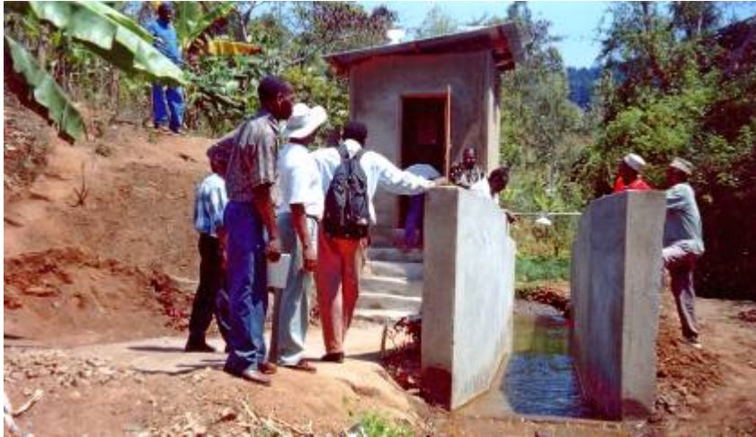
Figure 2.5: Flume at the outlet of the Tanzania catchment, plus cabin for equipment
