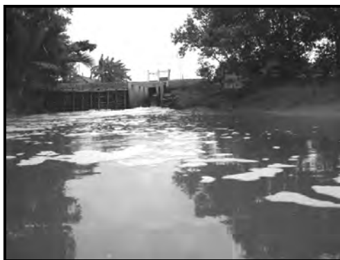
Water flowing out through a sluice gate. Shrimps and fishes are collected through a bag net put at this gate
