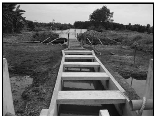
A concrete sluice gate in improved extensive farms
