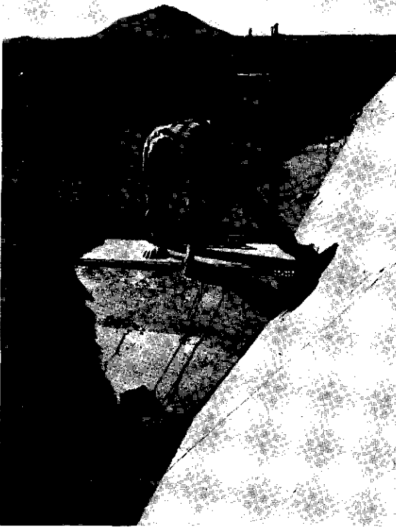
Photo 5.2. Temporary weir, custom-built of sheet steel
