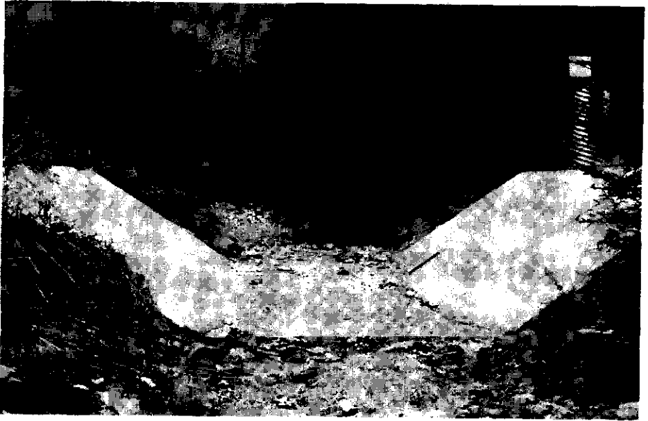
Photo 5.6. Flat-bottomed flume in the High School Wash, Tucson, Arizona
