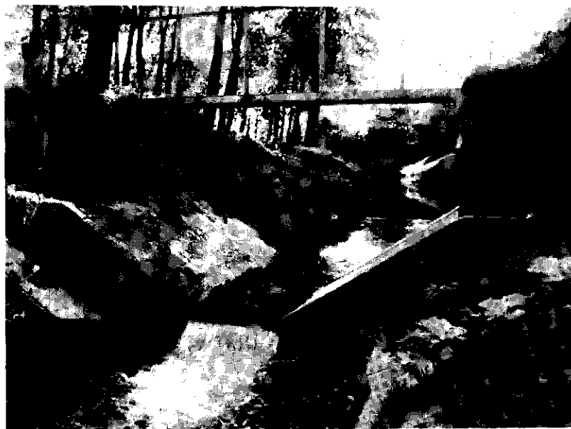
Photo 3.1. Long-throated flume with complex control section
