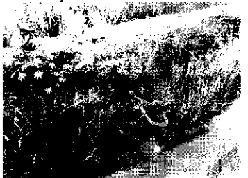
Photo 4.8: Staff of the Comisión is conducting a flow measurement with a current meter in the tertiary canal La Ladrillera
