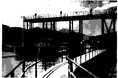
Photo 3.4: Main head work 'Botaza'
