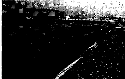
Figure 4.2. Typical trapezoidal concrete lined primary irrigation canal in Morocco: primary canal West in the Tessaout Amont irrigation system.
