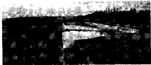
Figure 5.7. Sand trap at the head of the Primary Canal Ouled Gaid. With the present low water level, the silt deposits become visible.
