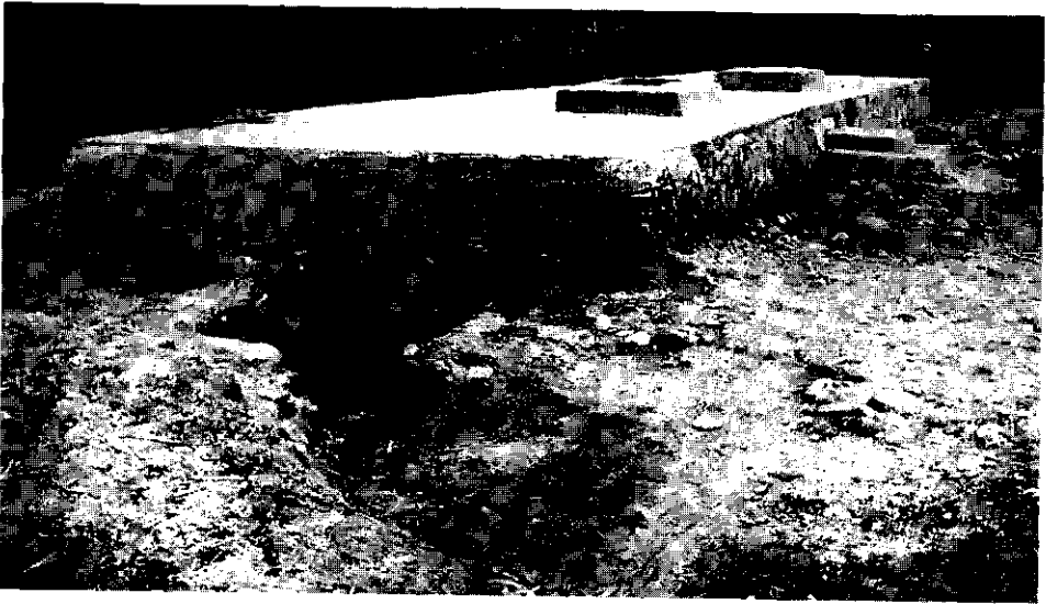
Figure 5.22. Communal metfia built with mud and stones and renovated with cement. The feeder canal that connects the secondary canal RG2 to the metfia has not been lined and is prone to pollution.
