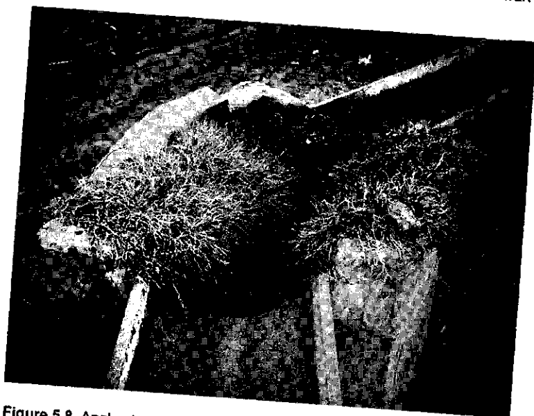
Figure 5.8. Angle structure at a tertiary canal, fully overgrown with weeds.
