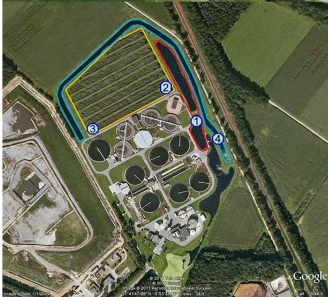
Figure 3 WWTP Land van Cuijk with constructed wetland compartments; sedimentation ponds (red frame), helophyte fields (yellow frame) and discharge ditch (blue frame). Numbers 1 to 4 indicate sampling positions.
