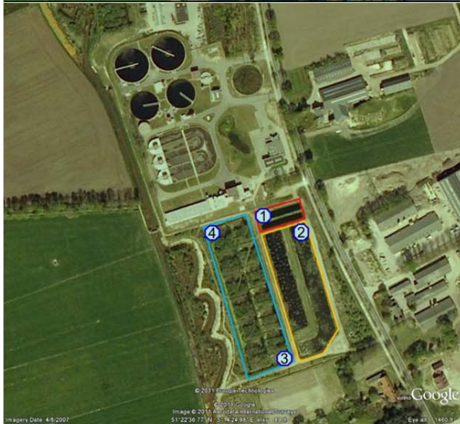
Figure 2 WWTP Hapert with constructed wetland compartments; sedimentation ponds (red frame), helophyte fields (yellow frame) and wetland forest (blue frame). Numbers 1 to 4 indicate sampling positions.
