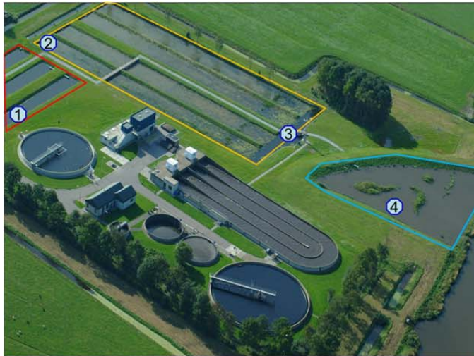
Figure 1 WWTP Grou with constructed wetland compartments; sedimentation ponds (red frame), helophyte fields (yellow frame) and ecological lagoon (blue frame). Numbers 1 to 4 indicate sampling positions.
