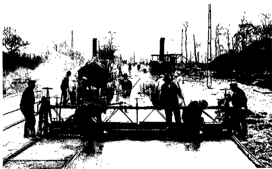
Following the United States and England in particular, asphalt and tar, in addition to bricks and concrete, played an increasing part in road construction. The mixture had to be processed after it had been heated, as we can see here during the construction of the Utrecht - De Bilt road around 1930
