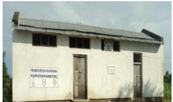
Photo 4: Store cum office building at ARC Betahani
