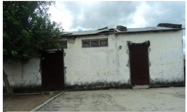
Photo 2: Store cum office building at ARC Khairapur
