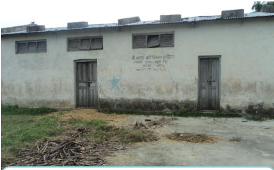
Photo 1: Store cum office building at ARC Machhagad
