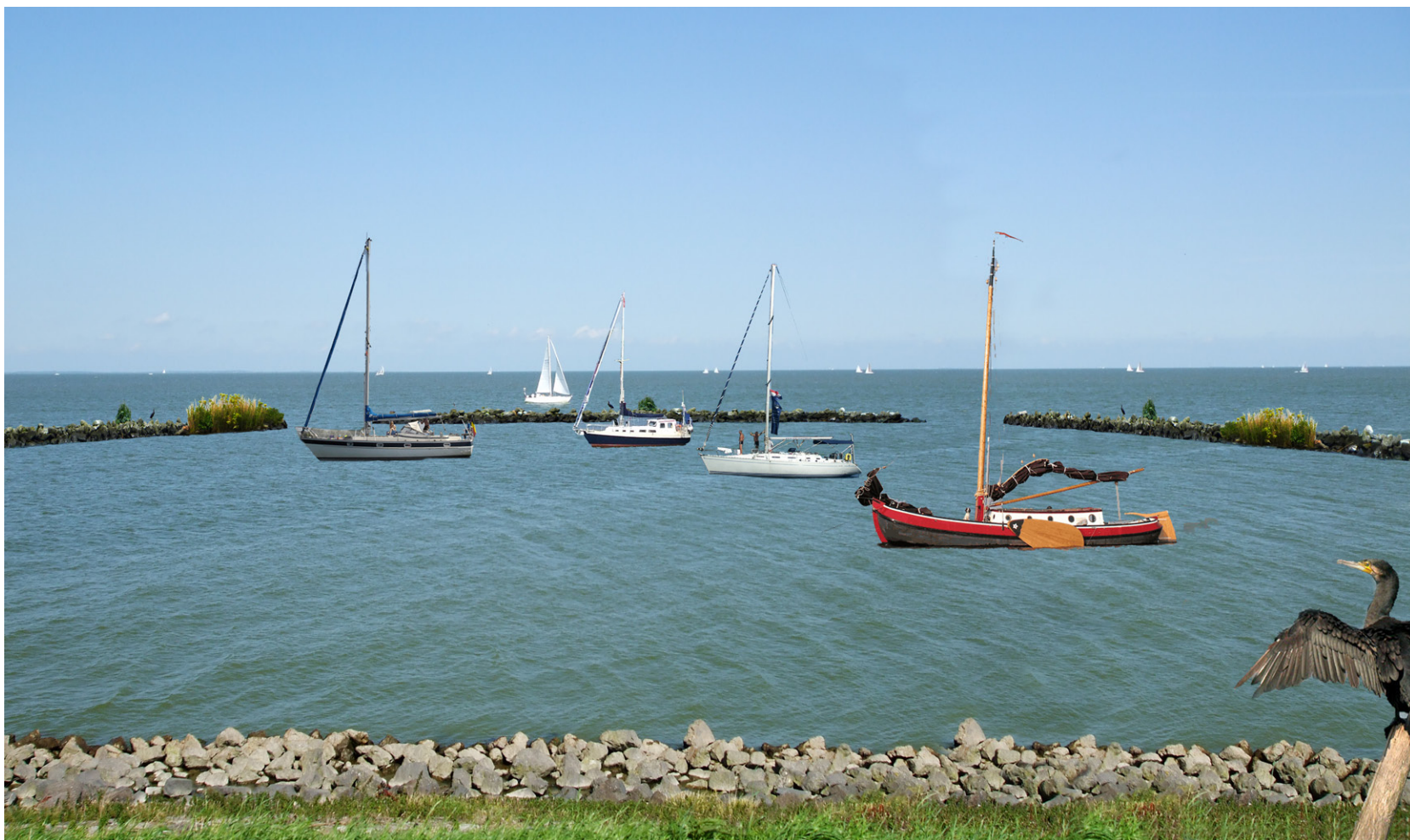
Figure 7.9a: visualisation of the anchorage area in front of the Zuiderzee museum. the shelter dams are kept low, and without high plant growth, so that the view from the museum towards the open water is not blocked. The area will offer a sheltered place for both traditional and modern boats. There also will be a jetty where ferry boats for the museum can land.
