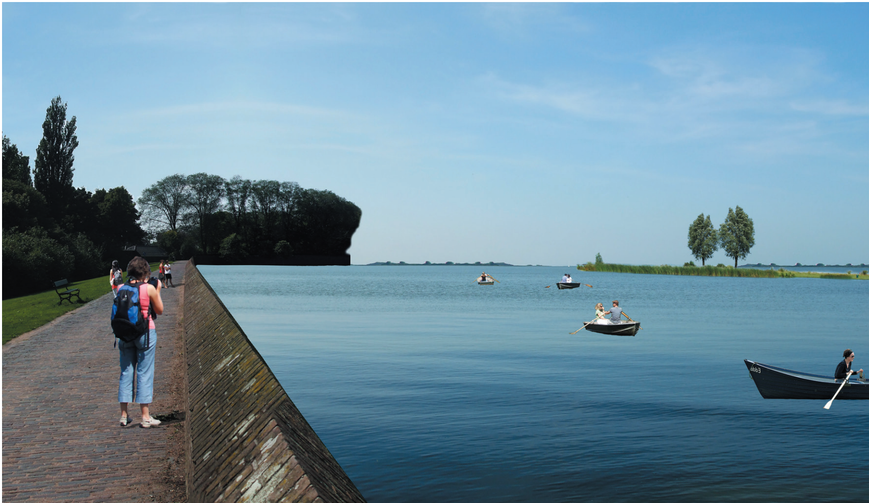
Figure 7.8a: visualisation of the new situation along the sea wall in Enkhuizen. The sea wall is again directly exposed to the water, so that its function is clear. The area in front of the dike which will not flood is visible nearby. On a distance the shelter dams, which are partly grown with plants, are visible.
