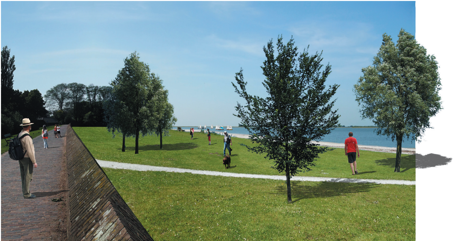
Figure 7.16a: visualisation of the new situation of the sea wall near Enkhuizen. The area in front of the wall will be redesigned, to create an open view from the wall to the water. The wall will not be exposed directly to the water, but it will be clear that it is a wall with a protection function. On a distance the new built dam is visible, and the area in between the wall and the dam is in use for all kinds of small scale watersports.
