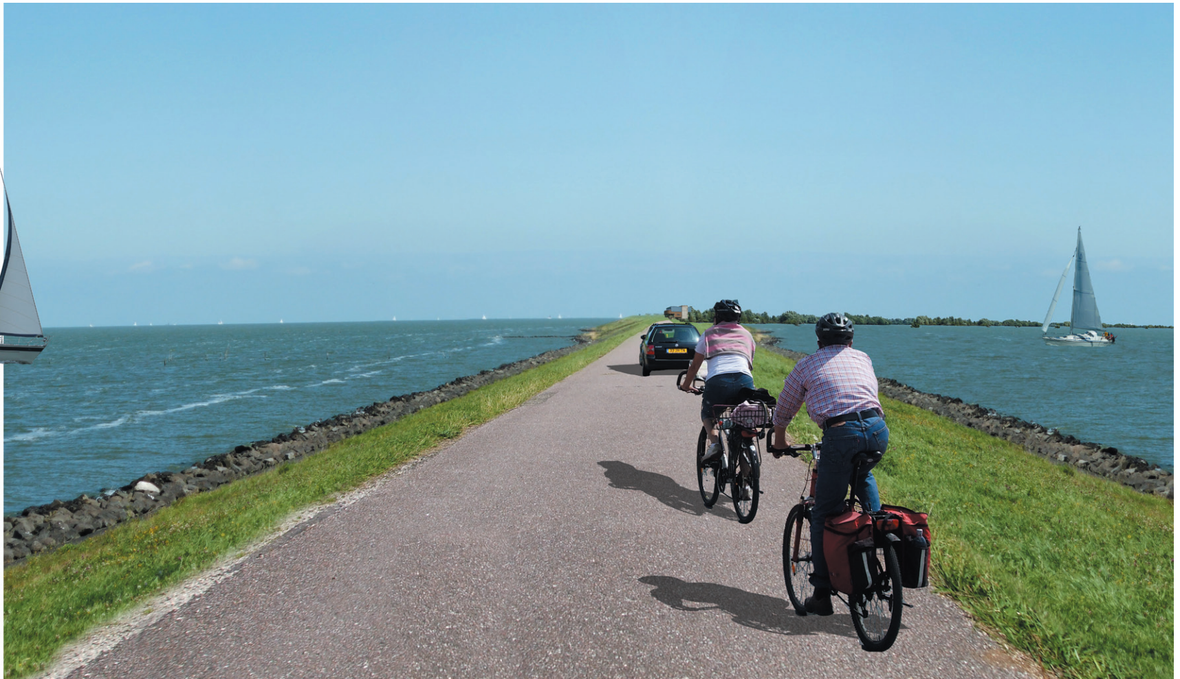
Figure 7.12a: visualisation of the narrow part of the new dam, from the Wieringermeer to the broad part of the dam. This part of the dam will be accessible for cars, also because the locks need to be accessible. On the left side the IJsselmeer is visible, on the right side it is the new created, sheltered lake which can be seen.
