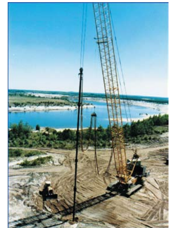
Picture 5.5: The rehabilitation of a former mine site, stabilization with 'Rütteldruckverdichtung'
