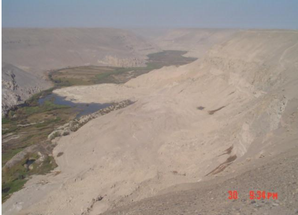
Photo 4.2: The water leak and the burying of Sihuas Valley's agricultural lands
