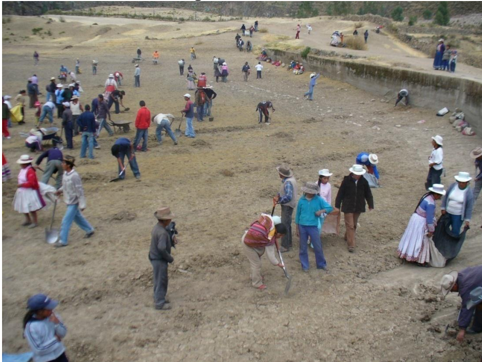
Photo 6.3: Cleaning of the reservoir Santa Rosa
