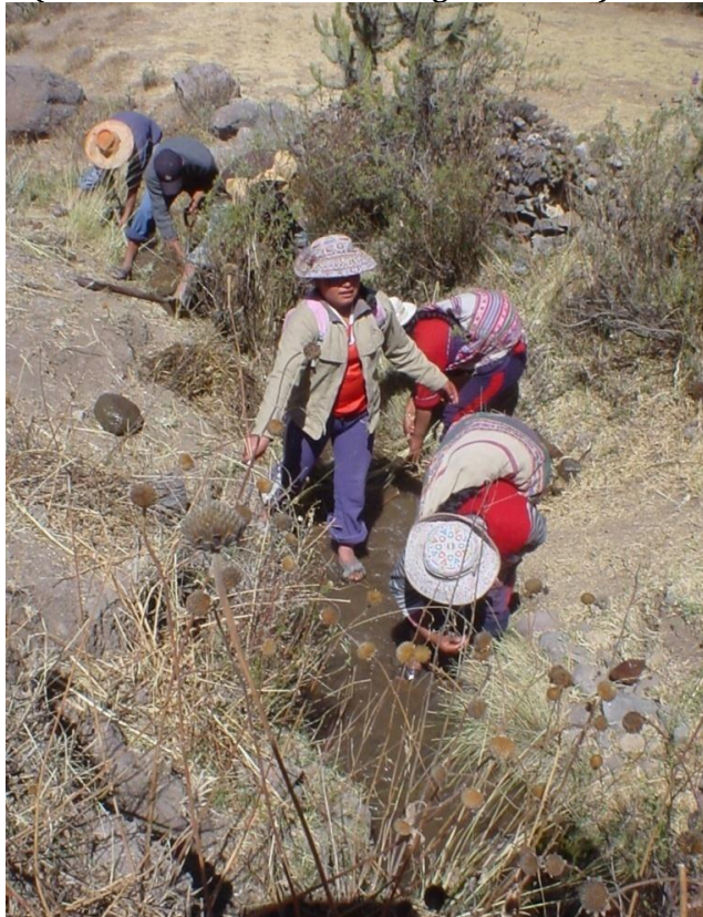
Photo 6.2: Cleaning of the canal (women head the work cutting the shrubs)
