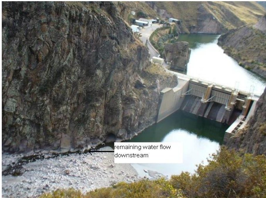
Photo 4.1: Reservoir-intake of MIP: Bocatoma de Tuti
