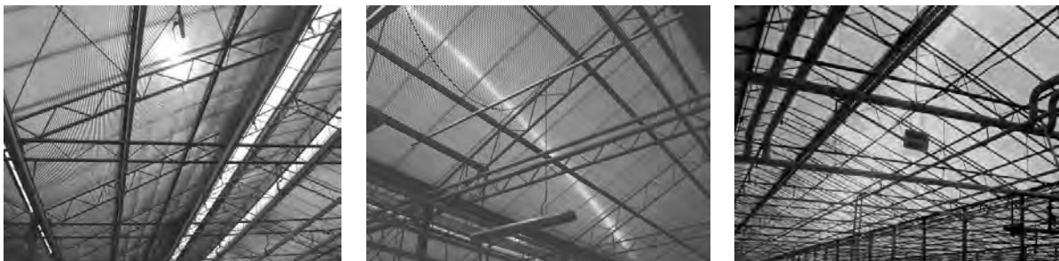
Figure 1. Photographs of the sun as it appeared in three compartments: glass (left), PC (middle) and PMMA (right). Note that screens are present in glass and PC, but absent in PMMA
