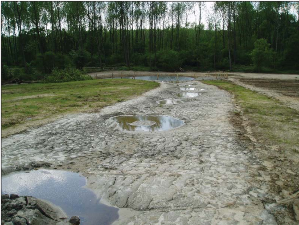
Figure 2. Wetland zone on wildlife overpass Groene Woud immediately after construction, consisting of a series of small ponds on loamy soils supplied by water that is pumped up to the top of the overpass (Photo courtesy of Rijkswaterstaat).
