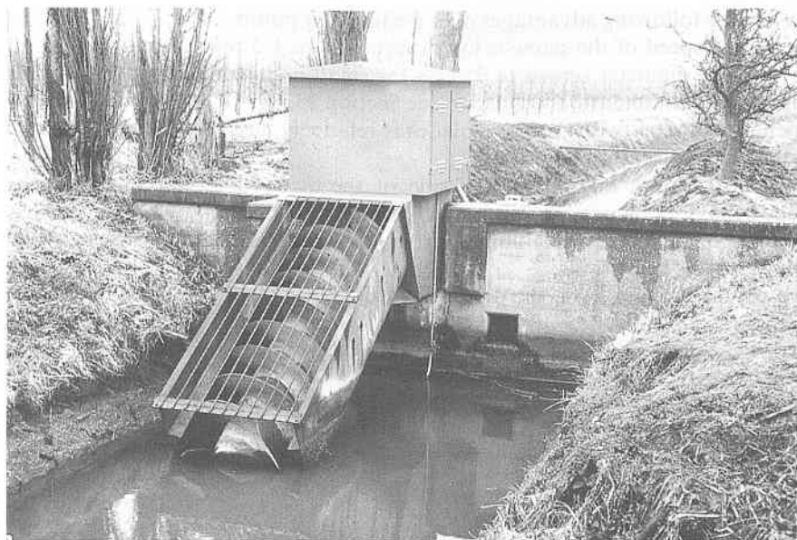
Photo 23.1 Small Archimedean screw in a drainage canal
