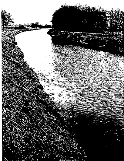
Photo 19.6 1980 Dec. 18 Some time after maintenance n = 0.040 (Courtesy University of Agriculture, Wageningen)
