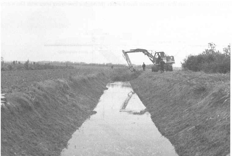
Photo 19.3 This machine can clean a drain with this top-width by working from one side only.
